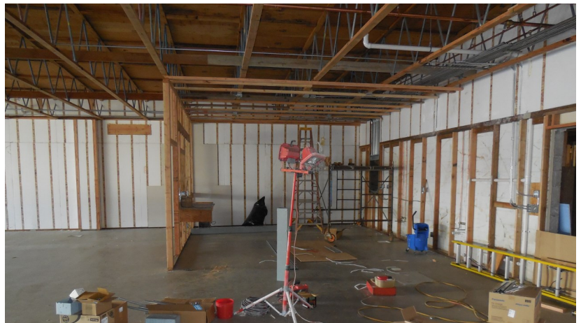
A view of the Kitchen framing after the wiring and before the drywall
