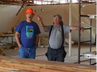
Richard & crew placed temporary supports through the center of the building before the roofing materials were delivered. When finished they will be removed.
